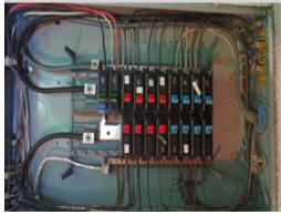
The electrical system of this home does not have a safe and effective way to quickly turn the power off in case of an emergency. Typically any system that requires more than six hand movements to shut down all system is considered unsafe. A licensed electrical contractor should be consulted for repair and a complete evaluation of the electrical system.
