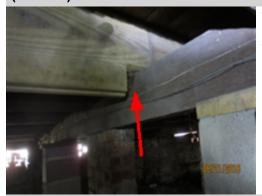
The floor joist located in the crawl space close to front of the home has been notched at the end. The notch is larger than what would be typically expected and could result in cracking or failure of the joist. A licensed general contractor should be consulted for further evaluation and to make necessary repairs.
