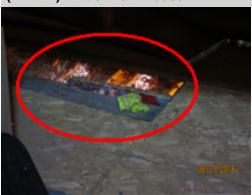
The soffit vents are covered or blocked. Improper ventilation could result in condensation, over heating of the building components, over heating of the building components, and inadequate conditioning of the living areas. A licensed general contractor should be consulted for repair/replacement.
