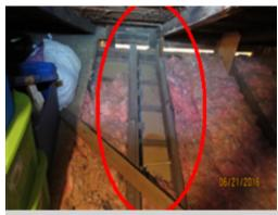
A section of insulation in the attic/ crawl space is missing. Improper insulation installation could result in condensation, over heating of the building components, and inadequate conditioning of the living areas. A licensed general contractor should be consulted for repair/ replacement.
