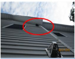
The siding for this home is a vinyl material. The siding on this home has visible areas of damage, cracking, mismatched colors, loose pieces, and fading. A licensed general contractor should be consulted for complete evaluation to locate and repair all areas of damage.
