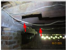
The floor joist located in the crawl space close to the front of the home has been notched. The notch is larger than what would be typically expected and could result in cracking or failure of the joist. A licensed general contractor should be consulted for further evaluation and to make necessary repairs.
