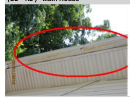
Additional Photograph: This is a photograph of rust on bottom, underside of gutter on the left side of main house near the back.
