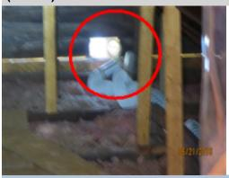
The bathroom ventilation fan exhaust duct does not exit to the exterior of the home. The fan exits to the attic space which will add undesirable moisture to the area. A licensed general contractor should be consulted for repair/ replacement.
