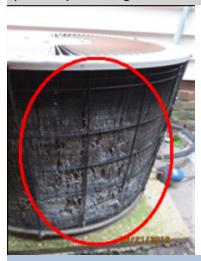
The outside compressor/coil unit for the heat pump system has visible damage to the coil fins. A damaged coil can result in leaking refrigerant and poor system performance. A HVAC contractor should be consulted for a complete evaluation and to make necessary repairs to ensure safe, reliable, and proper operation of the HVAC system.
