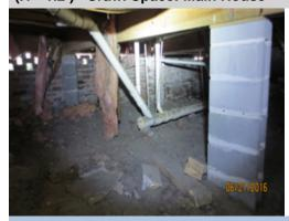
Additional Photograph: This is a photograph of wet insulation in crawlspace.
