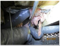
The insulation is/has been wet due to leaks or elevated area moisture levels. Typically insulation must be replaced if it has been because it does not retain fire protective coatings. The insulation needs to be replaced and the adjacent areas inspected for damage. See other sections for further information. A licensed general contractor should be consulted for repair/ replacement.
