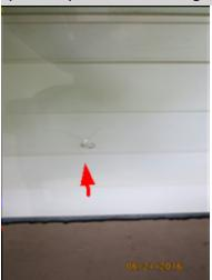
The siding for this home is a vinyl material. The siding on this home has visible areas of damage, cracking, mismatched colors, loose pieces, and fading. A licensed general contractor should be consulted for complete evaluation to locate and repair all areas of damage.
