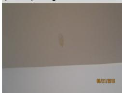
Stains on the ceiling in the main living room above front window indicate a history of a leak. At the time of the inspection it was not possible to determine if the condition was due to an active or past occurrence. Further investigation by a repair specialist and owner disclosure is recommended.
