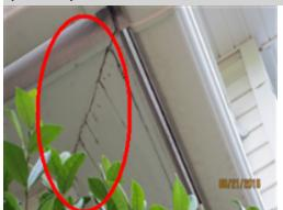
The roof gutters were found to be in poor condition and in need of repair /replacement. Evidence of roof drainage overflow in the boxing areas and behind the siding has resulted in visible areas of damage. Invasive inspection of boxing and adjacent siding areas is needed when gutters are repaired/ replaced. A licensed general contractor should be consulted for a complete inspection to determine the significance of the concern and to make necessary repairs.
